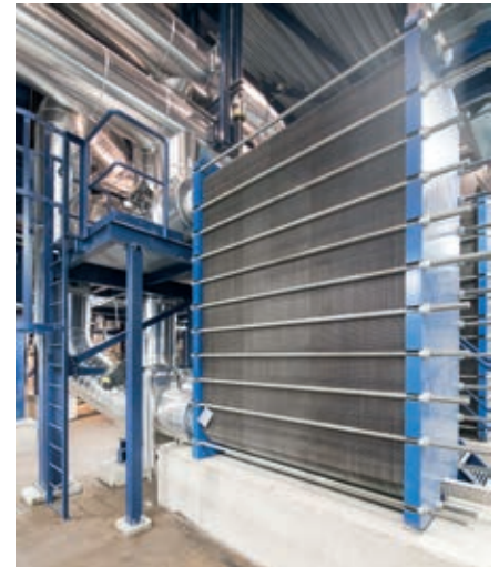
▲ Heat exchanger for transferring “waste” heat from the flue gas to the district heating network. Rauhalhti achieves 30-50 MW additional thermal energy with no increase in fuel consumption.
