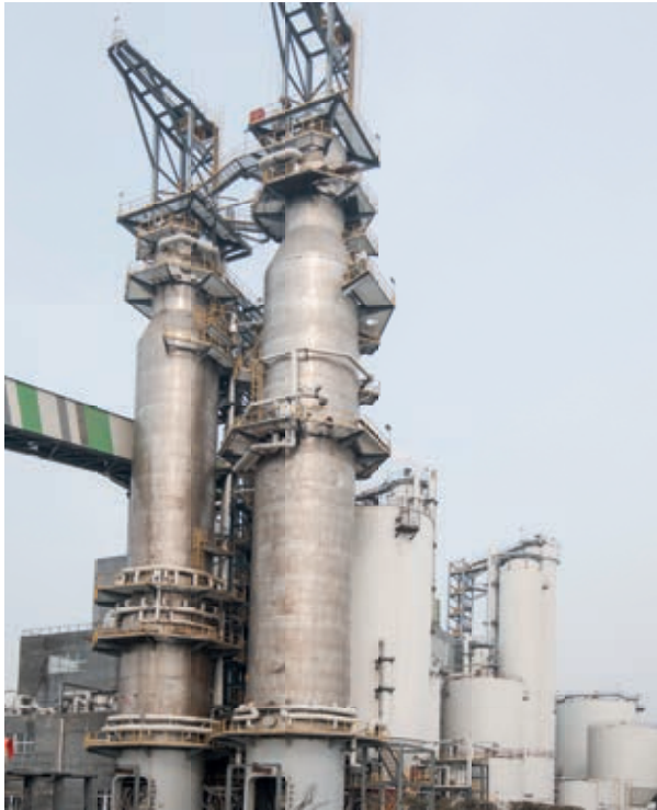
▲ The mill plans to swing between kraft and dissolving pulp depending on market demands and fiber availability. Twin vessels in the continuous cooking plant (a pre-hydrolysis vessel and a traditional digester vessel) make this flexibility possible.
