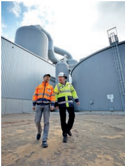
▲ Ronald Zierau, Project Manager for Zellstoff Stendal (left), walks through the upgraded evaporation plant with Tapio Lintunen, ANDRITZ Senior Project Manager.
