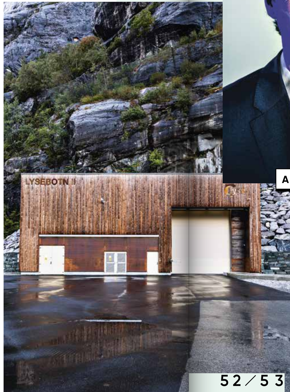
Entrance to the new Lysebotn II power station that went into operation in June 2018.
