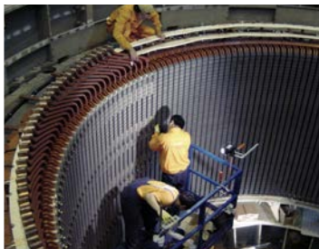
Drakensberg, South Africa 250 MW; Emergency repair, return to operation in minimum time
